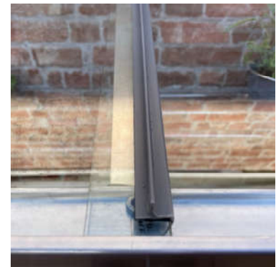
Roof glass overlapping
