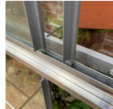
Glass in channel with two sheets overlapping
