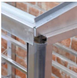
Corner trim in place
