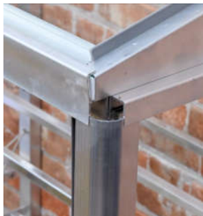
Corner trim in place
