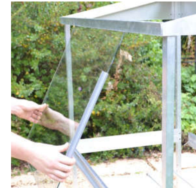
A. Fitting the glass
