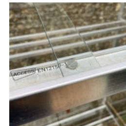
Roof glass overlap-
