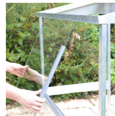
A. Fitting the glass
