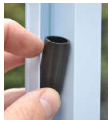
Fitting the hollow tube
