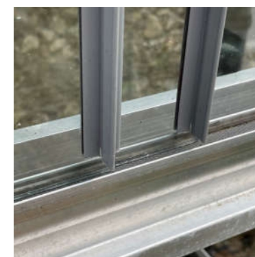
Glass in channel with two sheets overlapping
