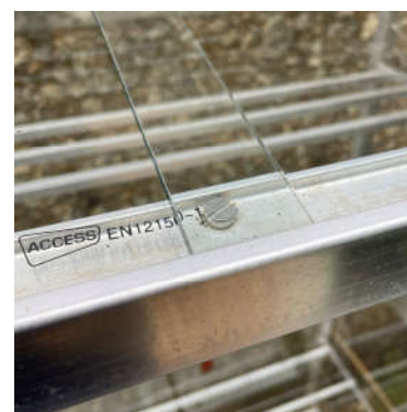
Roof glass overlapping
