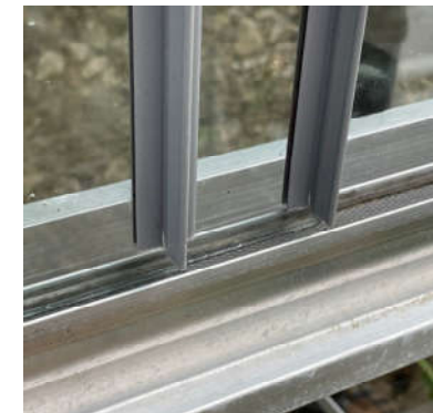
Glass in channel with two sheets overlapping
