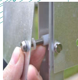
White spacers on infill plate
