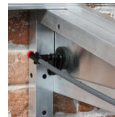
Inlet and link pipe
