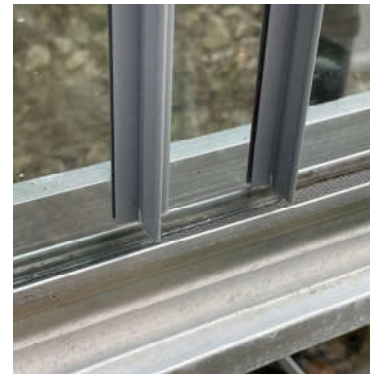
Glass in channel with two sheets overlapping
