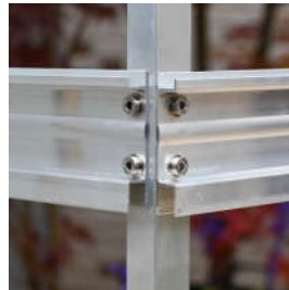
THE DEEPER CHANNEL GOES AT THE BOTTOM
