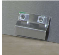
Completed bracket inside Growhouse
