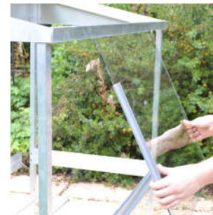
C. Fitting the glass
