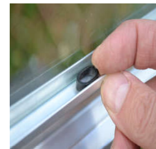
D. Ring wedge (Located in pack: SCREW-FB3)
