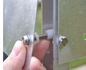
Nylon spacers on infill plate
