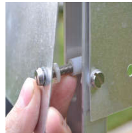
Nylon spacers on infill plate
