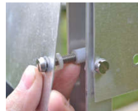
Nylon spacers on infill plate
