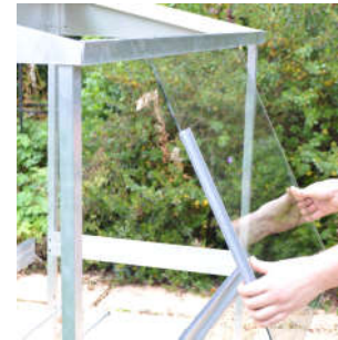
C. Fitting the glass
