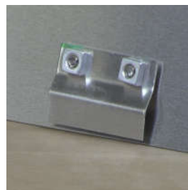
Completed bracket inside Growhouse
