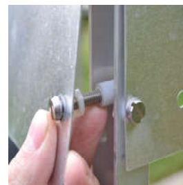
Nylon spacers on infill plate
