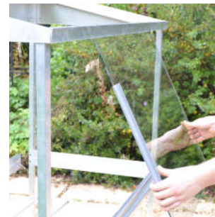
C. Fitting the glass
