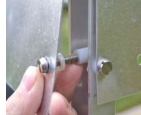
Nylon spacers on infill plate
