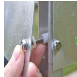
Nylon spacers on infill plate
