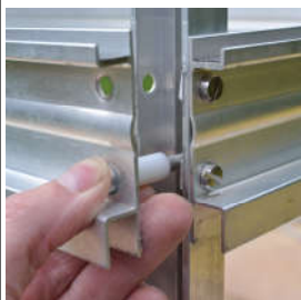
Nylon spacer on bolt
