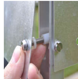
Nylon spacers on infill plate
