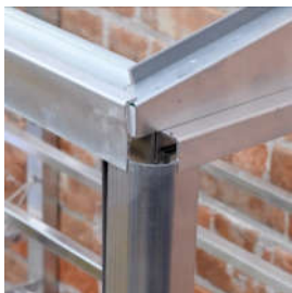
Corner trim in place
