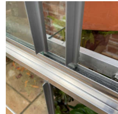
Glass in channel with two sheets overlapping
