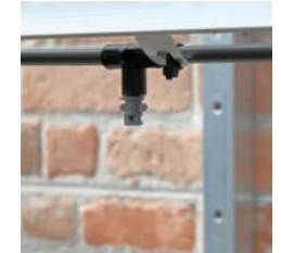
Nozzle strapped to 'L'
