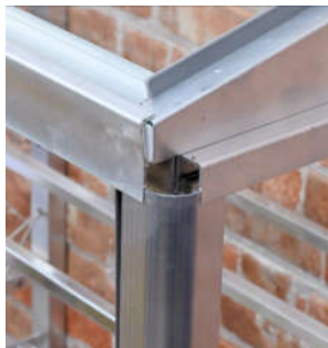
Corner trim in place
