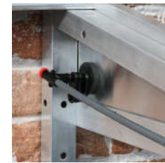
Inlet and link pipe
