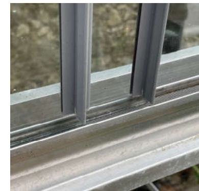
Glass in channel with two sheets overlapping
