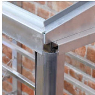
Corner trim in place
