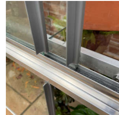
Glass in channel with two sheets overlapping
