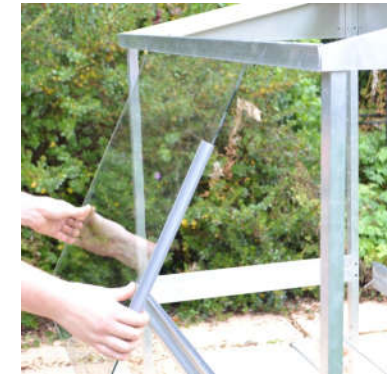
A. Fitting the glass
