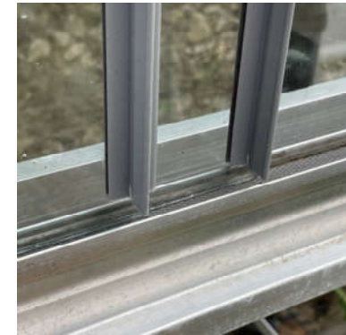
Glass in channel with two sheets overlapping
