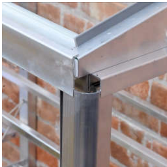
Corner trim in place
