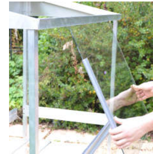
C. Fitting the glass
