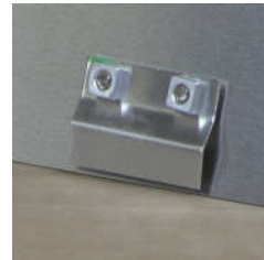
Completed bracket inside Growhouse
