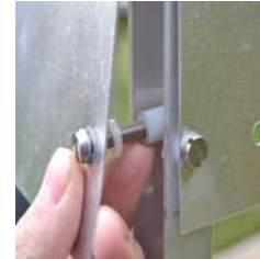
White spacers on infill plate
