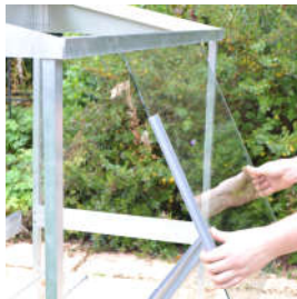
C. Fitting the glass
