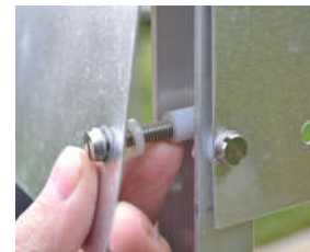
Nylon spacers on infill plate
