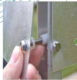
White spacers on infill plate
