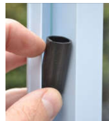
Fitting the hollow tube
