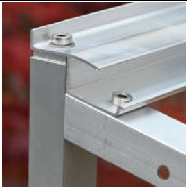
FIXING DETAIL
