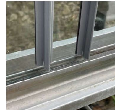
Glass in channel with two sheets overlapping
