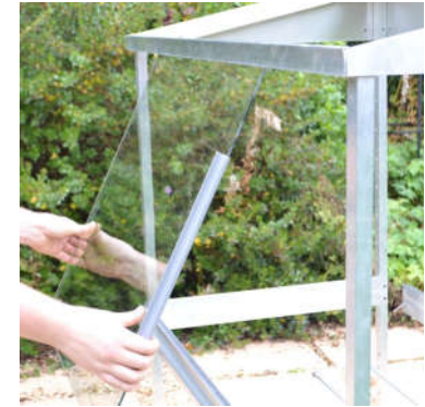
A. Fitting the glass
