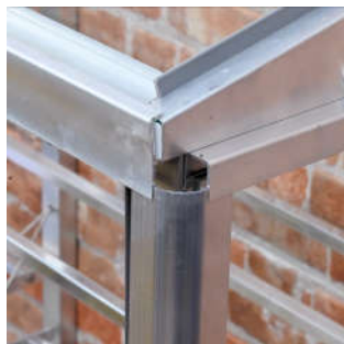
Corner trim in place
