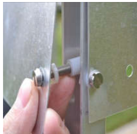
White spacers on infill plate
