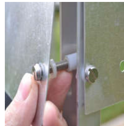
Nylon spacers on infill plate
