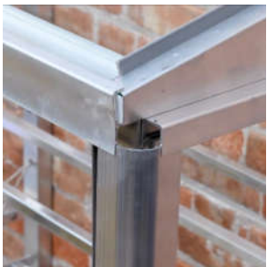
Corner trim in place
