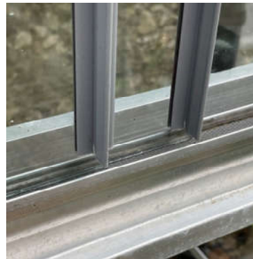
Glass in channel with two sheets overlapping
