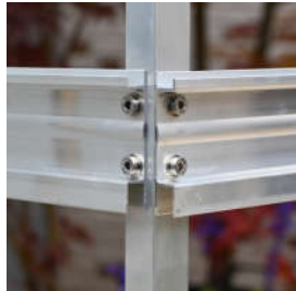
THE DEEPER CHANNEL GOES AT THE BOTTOM
