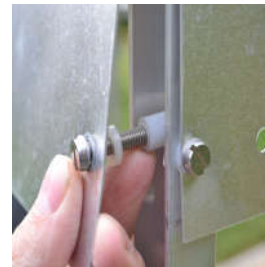
Nylon spacers on infill plate
