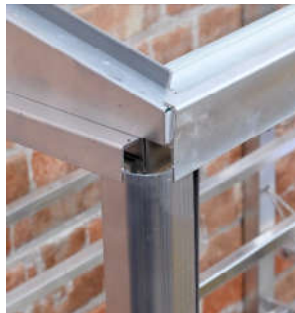
Corner trim in place
