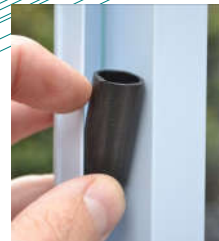
Fitting the hollow tube
