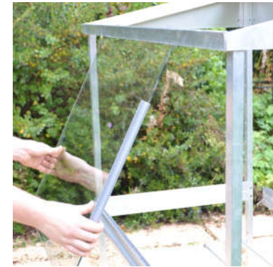
A. Fitting the glass
