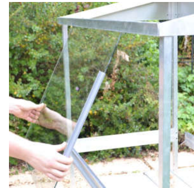
A. Fitting the glass
