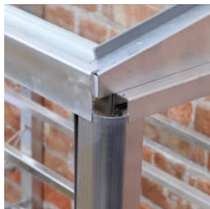
Corner trim in place
