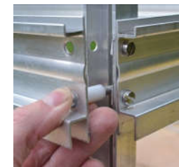
Nylon spacer on bolt
