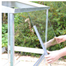
C. Fitting the glass
