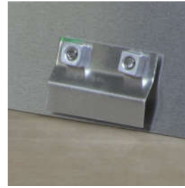
Completed bracket inside Growhouse
