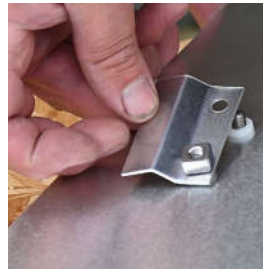
Nylon spacers on infill plate
