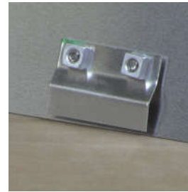
Completed bracket inside Growhouse
