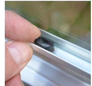
F. Ring wedge (Located in pack: SCREW-H9 )
