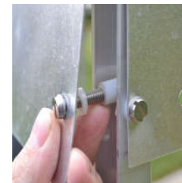
Nylon spacers on infill plate
