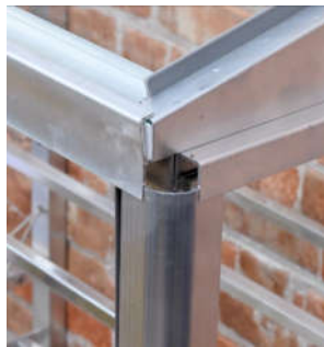
Corner trim in place
