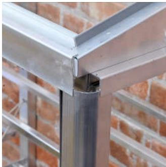
Corner trim in place
