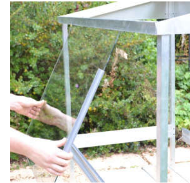
A. Fitting the glass
