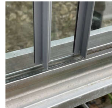
Glass in channel with two sheets overlapping
