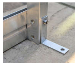
ANCHORAGE BRACKET FITTED
