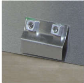
Completed bracket INSIDE Growhouse
