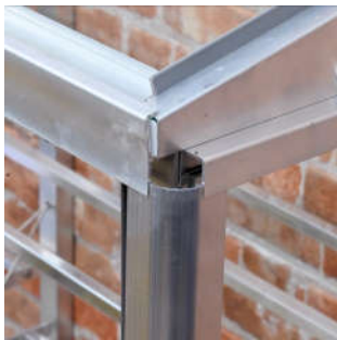
Corner trim in place
