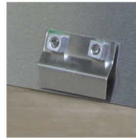
Completed bracket inside Growhouse
