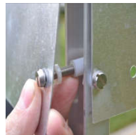
Nylon spacers on infill plate
