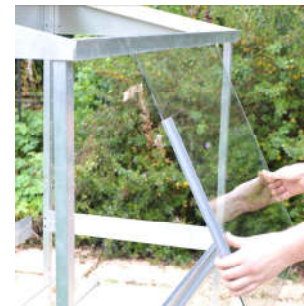
C. Fitting the glass
