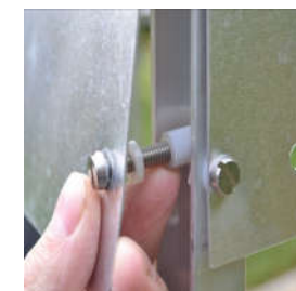
Nylon spacers on infill plate
