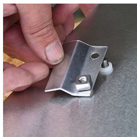
Nylon spacers on infill plate
