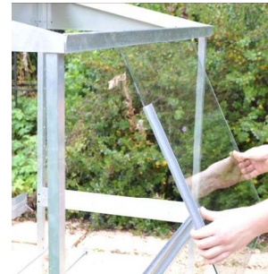
C. Fitting the glass
