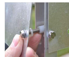
White spacers on infill plate
