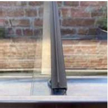
Roof glass overlapping
