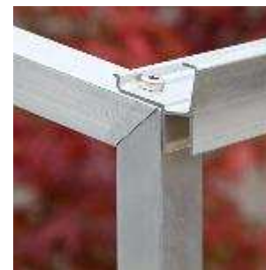
IMAGE 4 No gap in mitre and front top rail fitted properly
