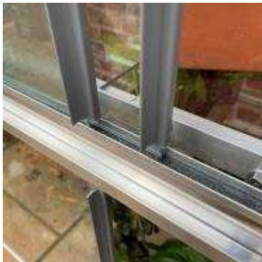
Glass in channel with two sheets overlapping
