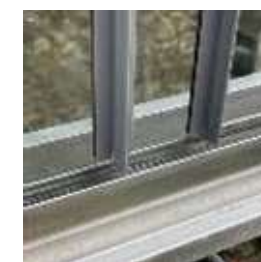
Glass in channel with two sheets
