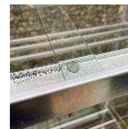
Roof glass overlapping
