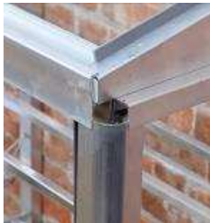
Corner trim in place
