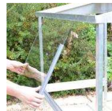
A. Fitting the glass
