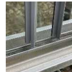
Glass in channel with two sheets overlapping
