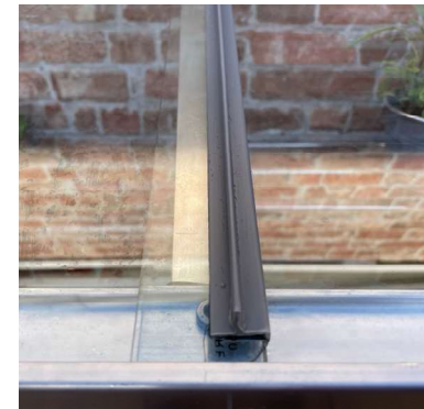
Roof glass overlapping
