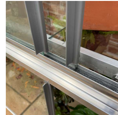
Glass in channel with two sheets overlapping
