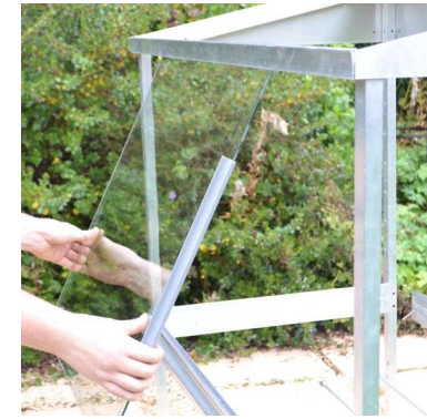
A. Fitting the glass
