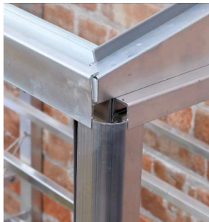
Corner trim in place
