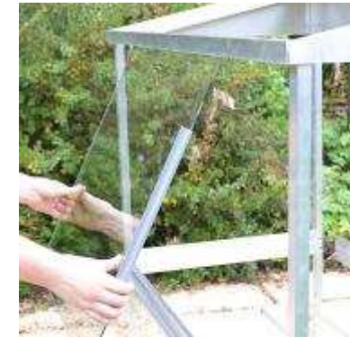
A. Fitting the glass
