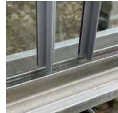
Glass in channel with two sheets overlapping
