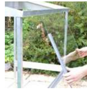
C. Fitting the glass
