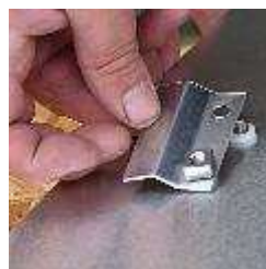
white spacers on infill plate
