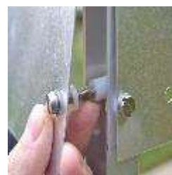
Nylon spacers on infill plate
