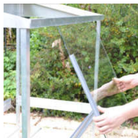
C. Fitting the glass
