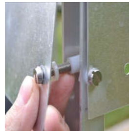
Nylon spacers on infill plate
