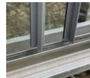
Glass in channel with two sheets overlapping
