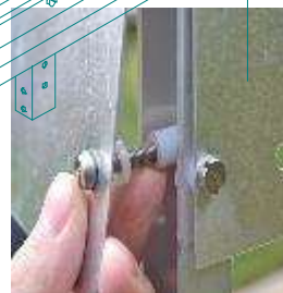
White spacers on infill plate
