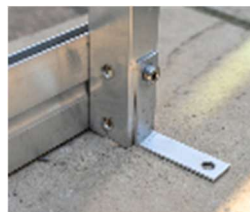
ANCHORAGE BRACKET FITTED
