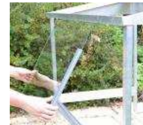
A. Fitting the glass
