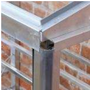
Corner trim in place
