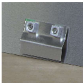
Completed bracket inside Growhouse
