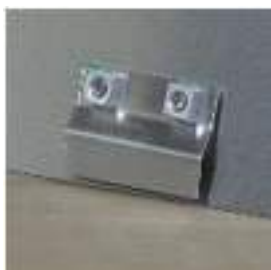
Completed bracket INSIDE Growhouse
