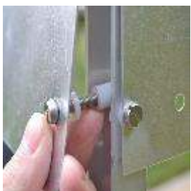
Spacers on infill plate
