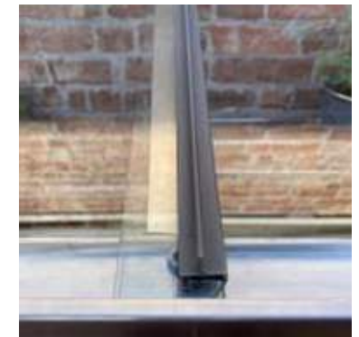
C. Roof glass overlapping
