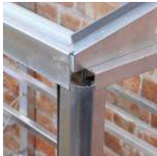
Corner trim in place
