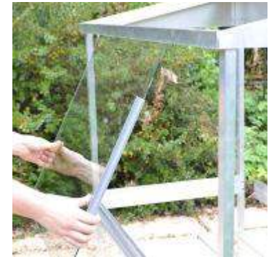
A. Fitting the glass
