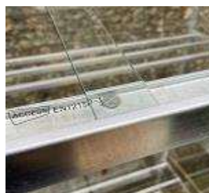
Roof glass overlapping
