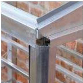
Corner trim in place
