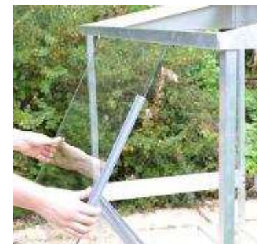
A. Fitting the glass
