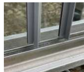
Glass in channel with two sheets overlapping
