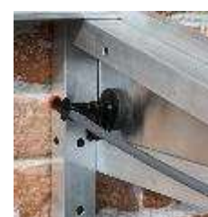
Inlet and link pipe
