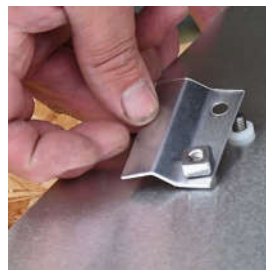
Nylon spacers on infill plate
