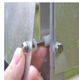
Nylon spacers on infill plate
