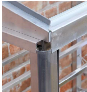
Corner trim in place
